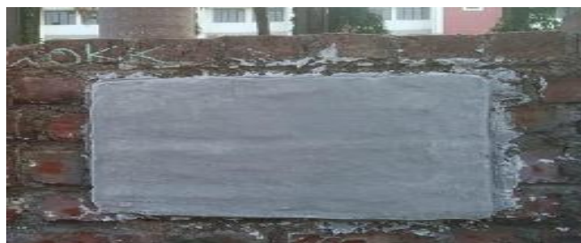
Figure 9: Eco Plaster Application
